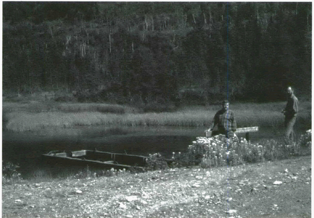
Special construction measures for a road crossing a marshy creek. The road bed is an earth fill dam which raises the water level to enhance the wetland for waterfowl habitat. A fish pass structure is in the middle of the photo.
