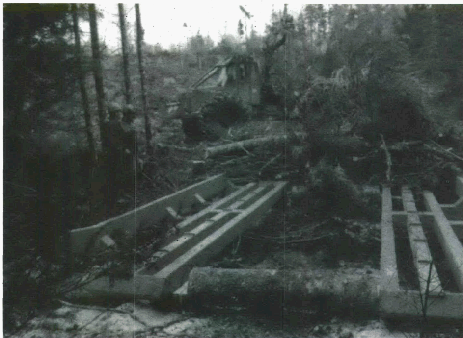
Portable steel bridges are one method of stream protection in forwarder operations.
