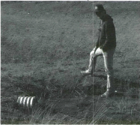
A cross-drain culvert installed to direct drainage under a road bed. Note the berm constructed behind the culvert to control drainage along the right-of-way.
