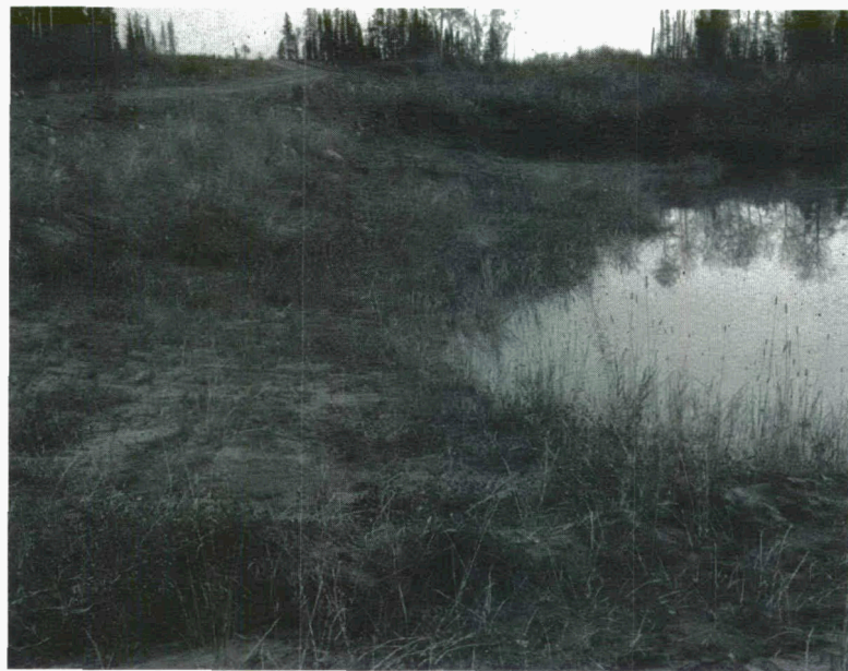
A sediment pond maintains water quality for runoff from a road.
