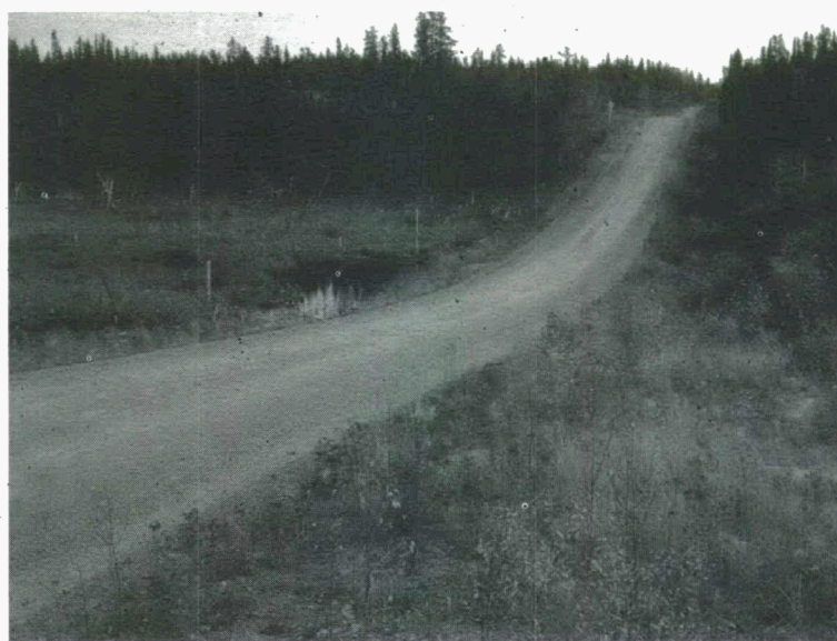
A forest road restricting drainage, causing flooding on the upstream side.
